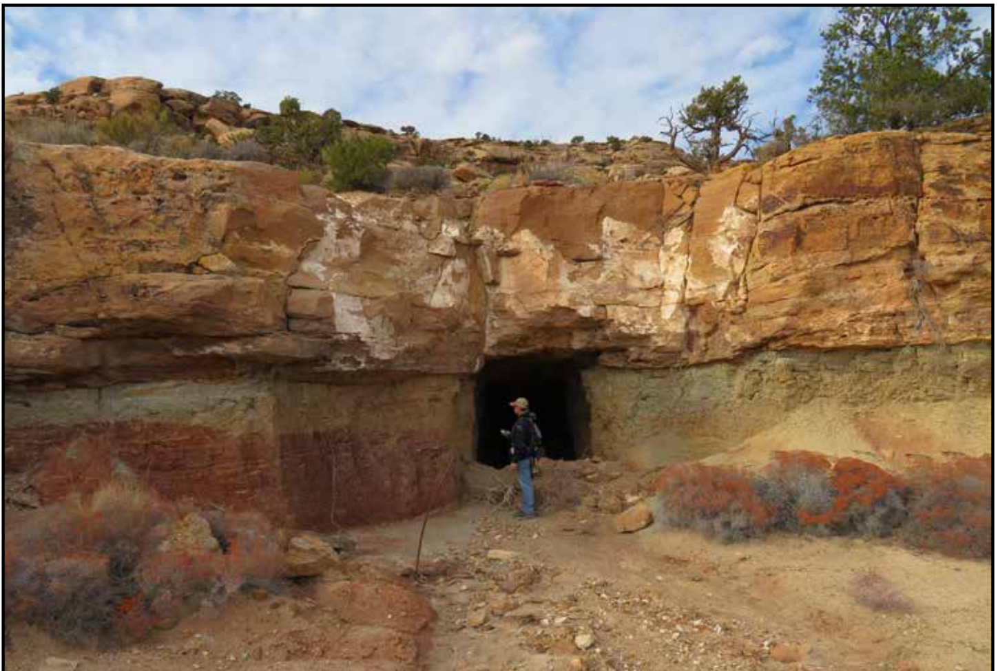
Uracop 3 Mine adit with sloughing in portal, Red, White and Fry Canyons and Deer Flat Districts, Utah, BLM-administered public land.
