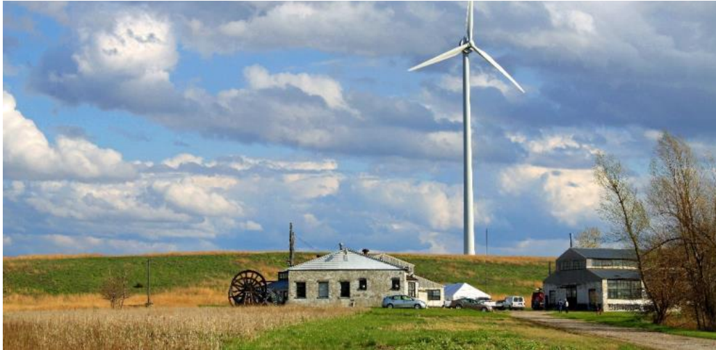
The Gob Nob wind turbine in Farmersville, IL is located on the former Freeman United Crown Number 1 Coal Mine. Photo from RECC.
