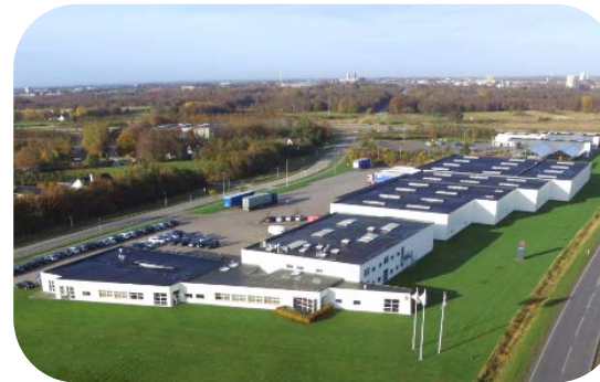
Denmark (Herning) H 2 Fueling Stations
