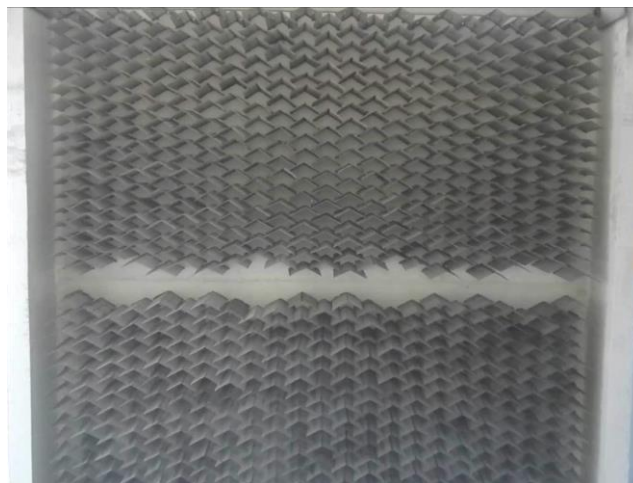
Obstructed Flow (KSU, GT)
