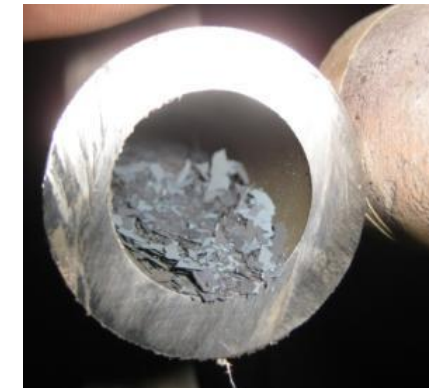
Exfoliation Blockage & Damage in New SC Coal and Combined Cycle HRSGs (Design & Materials)
