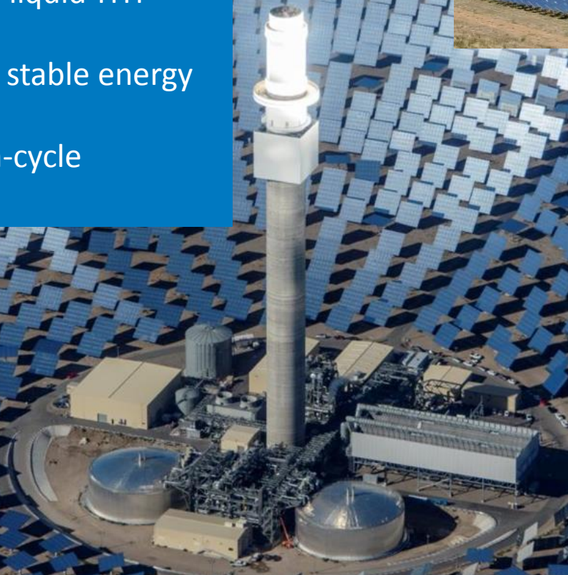
SolarReserve's Crescent Dunes molten-salt HTF, Nevada, USA
