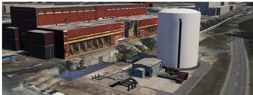
The “Headworks” component of the Outfall 200 Mercury Treatment Facility
