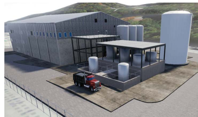
The “Treatment Plant” component of the OF200 MTF
