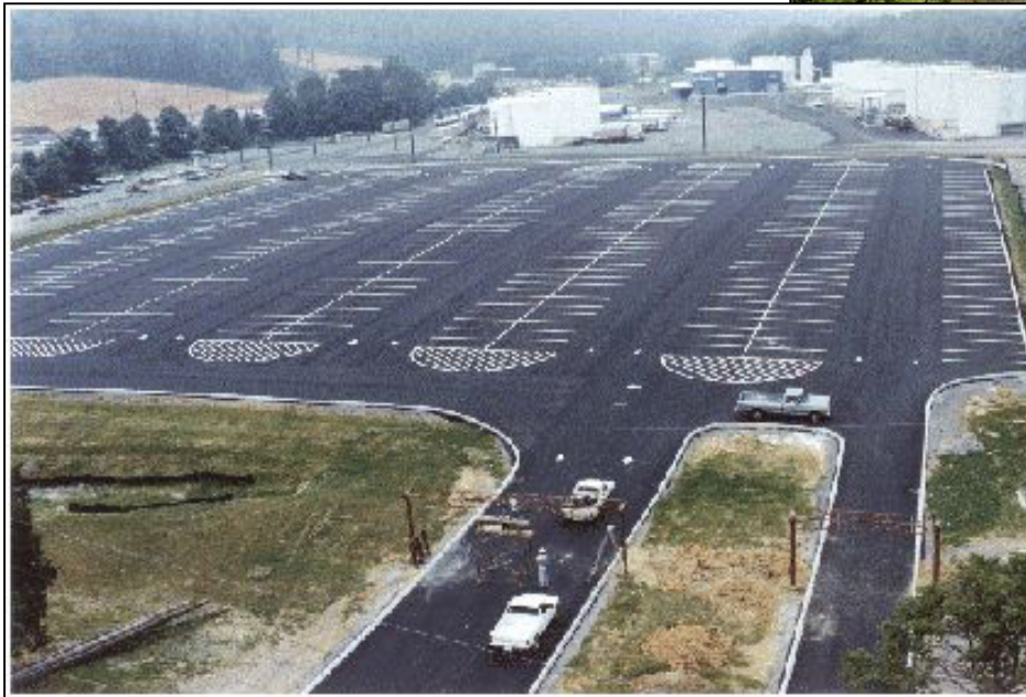
A parking lot now covers the old S-3 Ponds site
