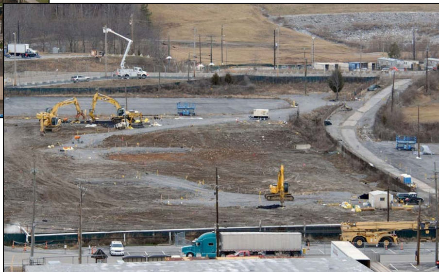
Y-12 Salvage Yard as cleanup neared completion
