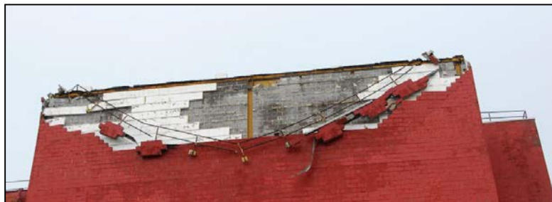
Bricks falling off the walls made demolition imperative
