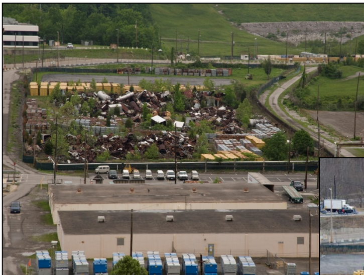
Y-12 Salvage Yard at the beginning of the project
