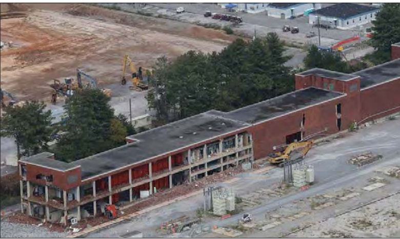
Building K-731 during demolition.
