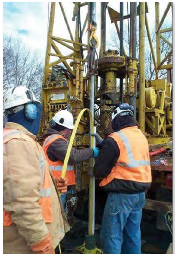
Monitoring wells were drilled on the west side of the Clinch River to determine if any contamination was migrating from DOE property into groundwater on private property
