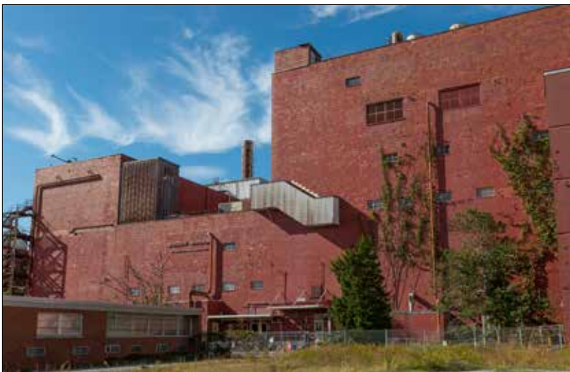
The Biology Complex is one of Y-12's excess contaminated facilities. Characterization has been completed to identify contaminants and prepare it for demolition and disposition.
