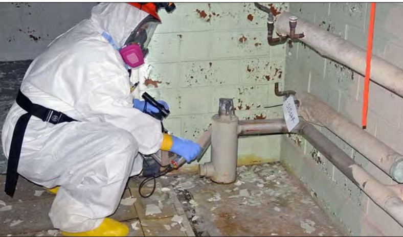
A technician surveys a pipe inside one of the buildings in the Biology Complex for contamination.
