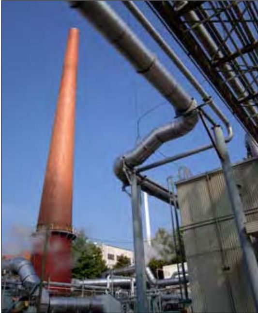
ORNL's Central Stack is part of an aging ventilation system that has reached the end of its usefulness.
