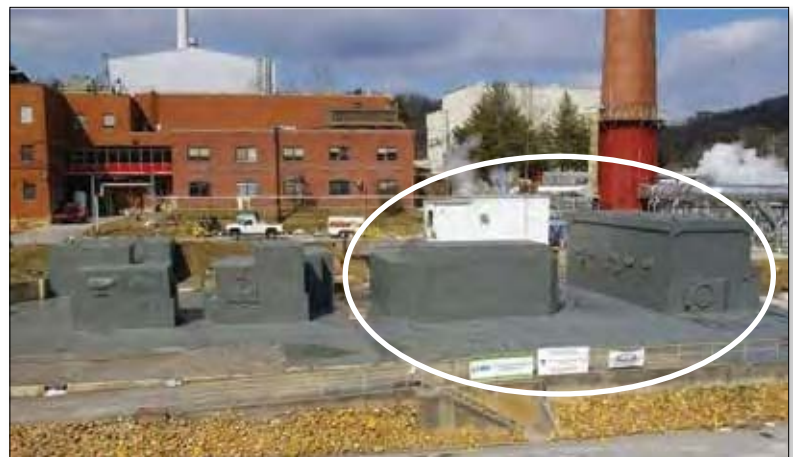
Two hot cells (circled) from Building 3026, remain from building demolition and require eventual disposition. The others have been removed.
