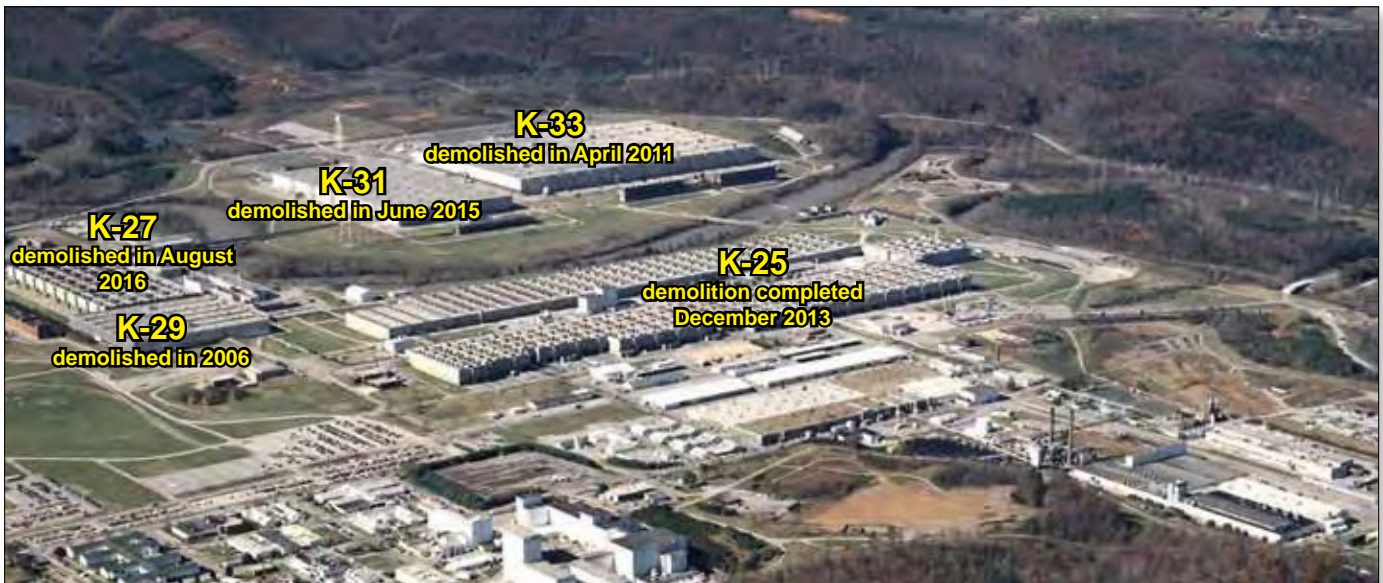
The K-25 Gaseous Diffusion Plant was renamed East Tennessee Technology Park in 1997. The goal is to clean up the area sufficiently so it can be turned into a private industrial park. This is how the site looked before major demolition work began.
