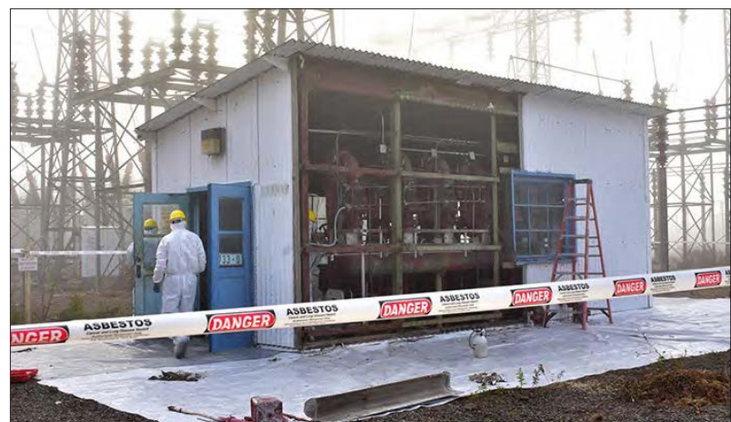
CTI workers clean up the K-732 switchyard
