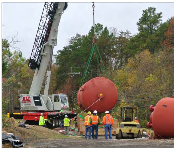
One of the five mercury tanks is excavated for disposal in 2013
