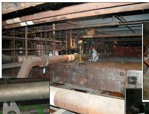
Left: sampling process systems in K-25
