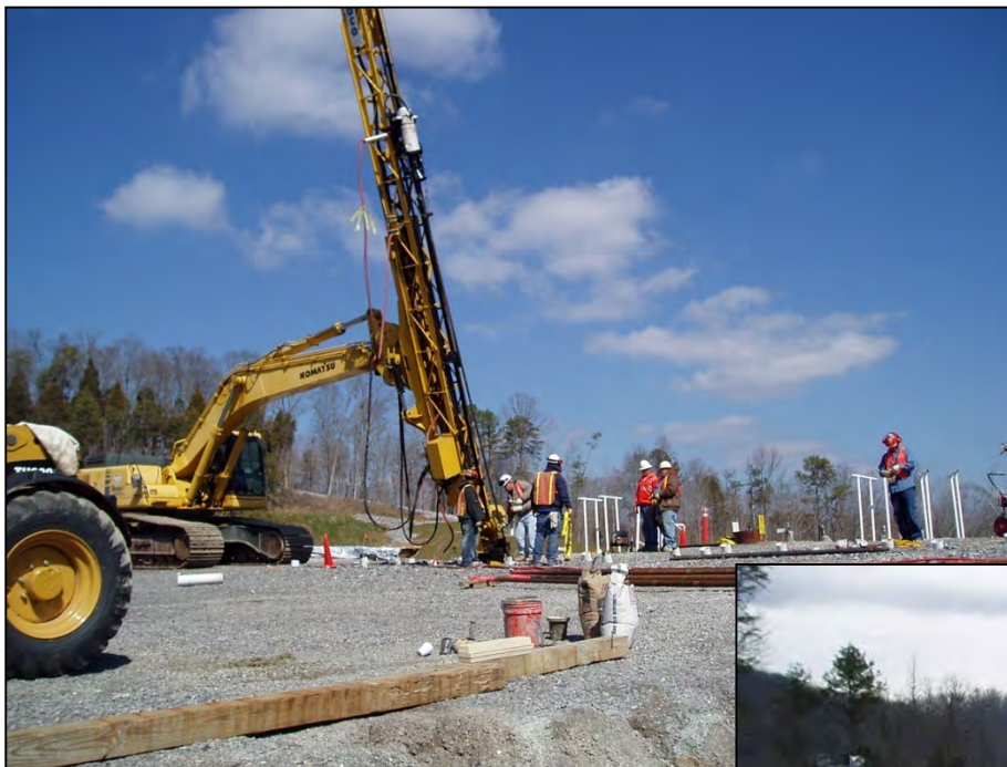
Driving sleeve pipes to inject grout at Trench 7
