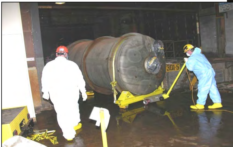
Converter prep for shipment for disposal
