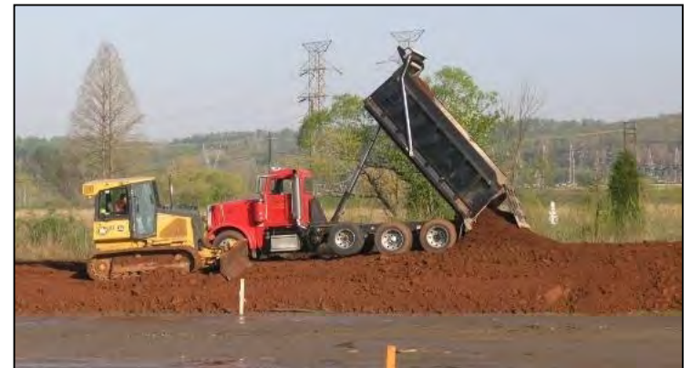
Clean fill being placed over PCB-contaminated sediment
