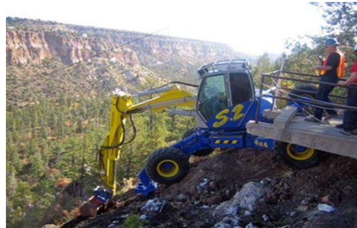
Spider Excavator on Canyon Edge
