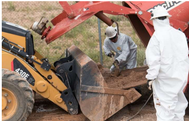
PCB contaminated soil removal TA-61
