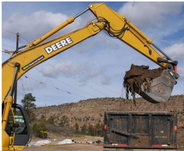
North Ancho Remediation
