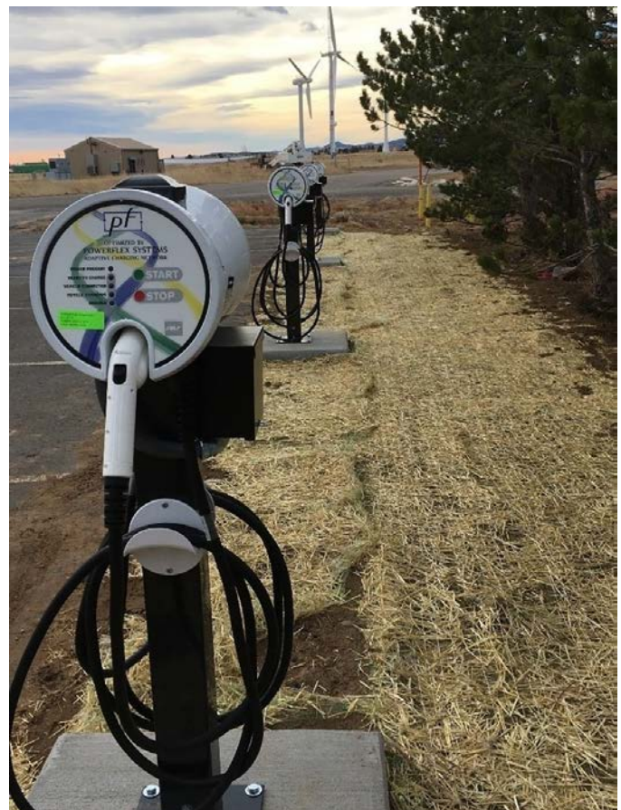
Erosion control blanket and underlying native seed surrounding electric car charging stations; the stations were installed as part of a research project to test equipment function and durability.
