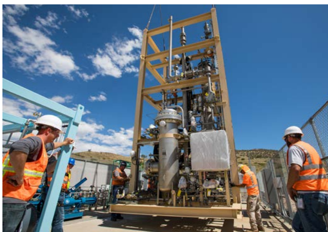
Crews work to install the first power-to-gas system in the U.S. at the STM site. Southern California Gas partnered with NREL on the project, which takes excess electricity and converts it to hydrogen, which can be used, stored or combined with carbon dioxide to produce renewable natural gas. Photo by Werner Slocum, NREL 47256
