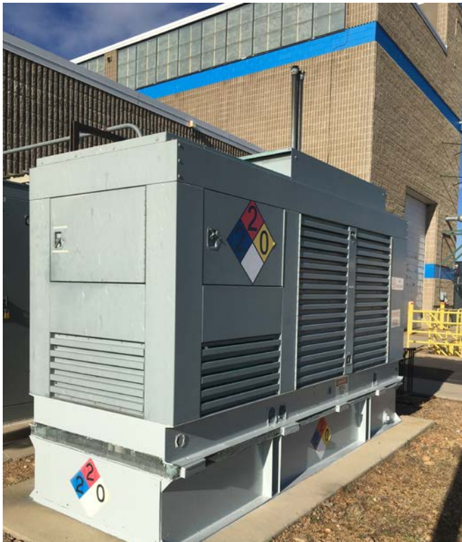
A double-wall 200-gallon (757-liter) standby generator diesel fuel tank located at the NWTC. Photo by Theodore DeVito NREL 50079
