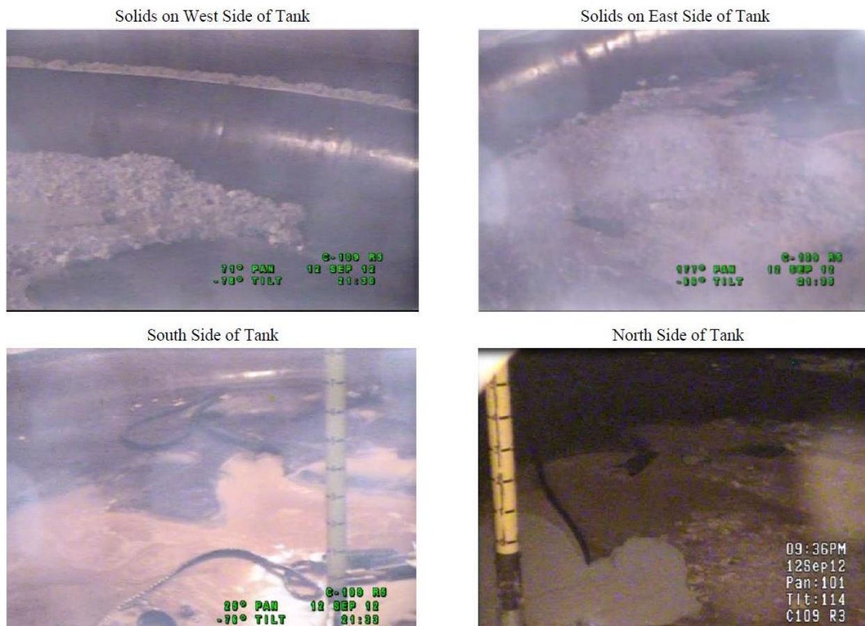
Figure 4-20. Photographs of Tank C-109 at Completion of Caustic Cleaning.
