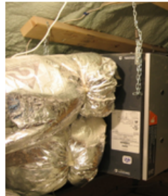
This HRV, installed in a c provides balanced ventil home
