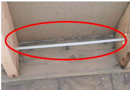
Bottom plate/sheathing gap
