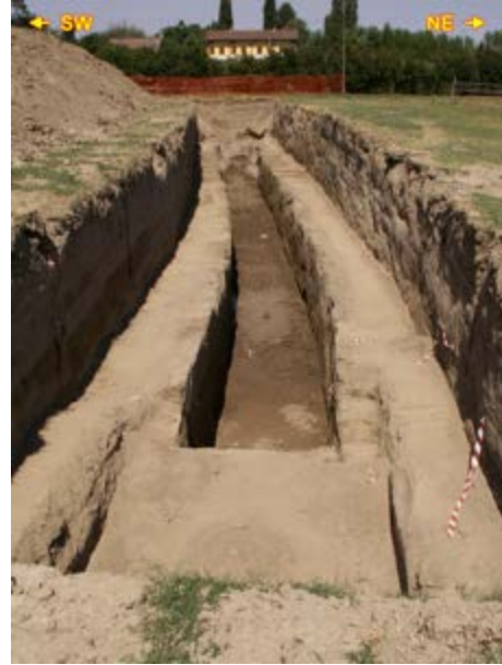
Benching Stabilization
