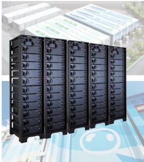
Energy Storage System
