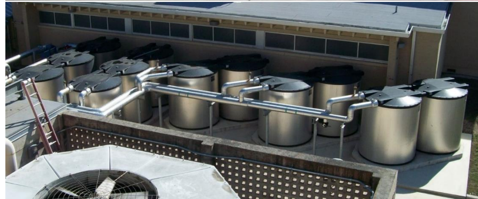
Fossil Ridge High School, Fort Collins Thermal Ice Storage System
