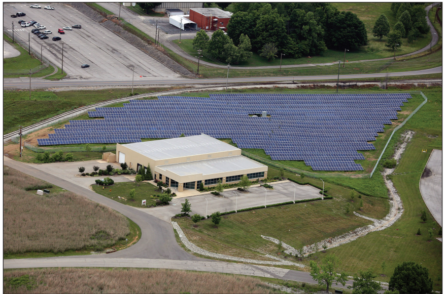
The Powerhouse Six solar array began operating at ETPP in 2015. It is a 1 megawatt power-generating facility located on a five-acre parcel and generates around 1.4 million kWh annually.
