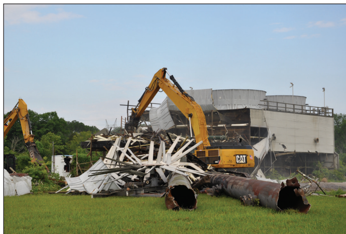
K-832-H Cooling Tower demolition.
