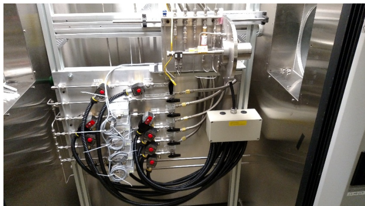
Figure II-376. Burner Hood with Cabot Inspired Burner
