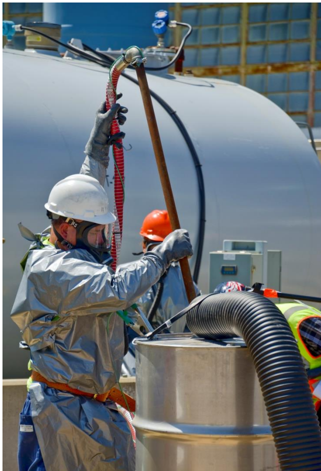
A technician pumps TCE from a storage tank (background) to containers
