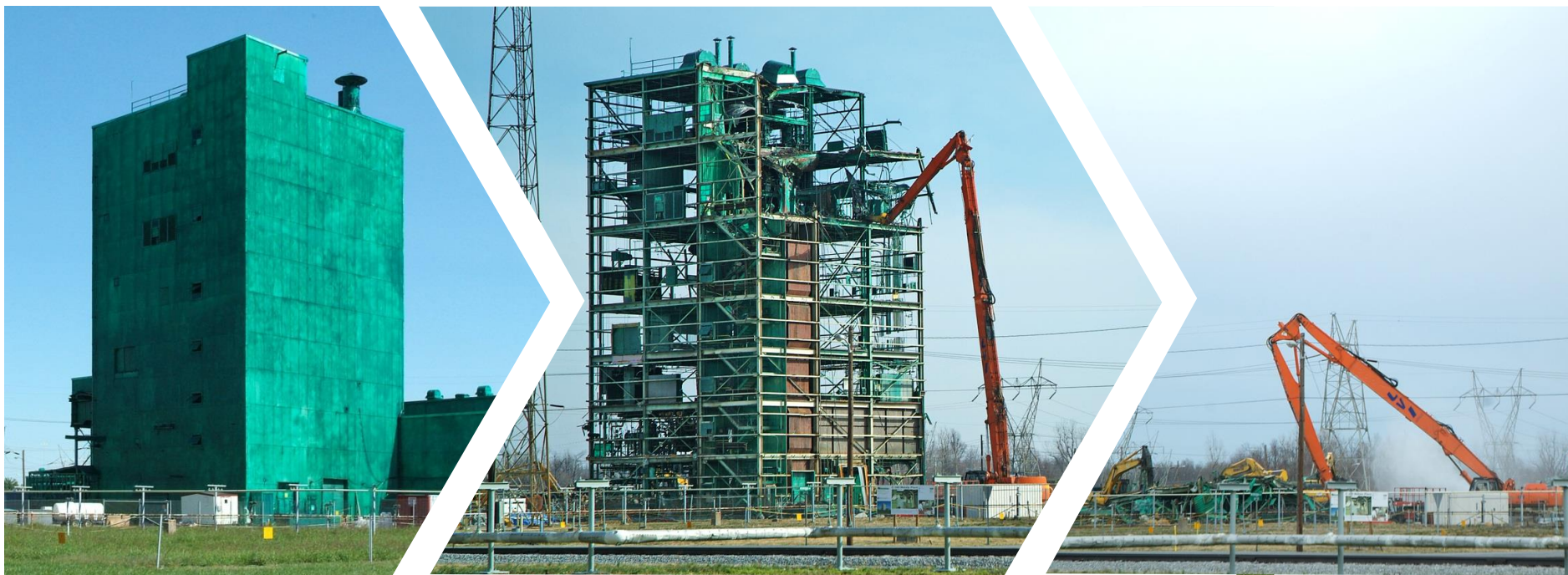
Progress of the demolition of C-340 Metals Plant
