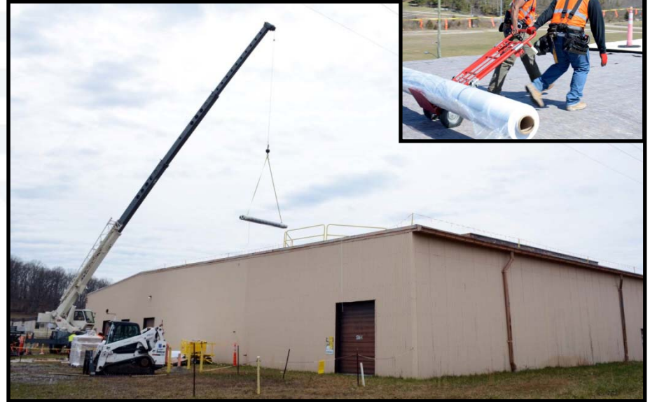
Above, an off-road crane was used to lift supplies for the crew.
