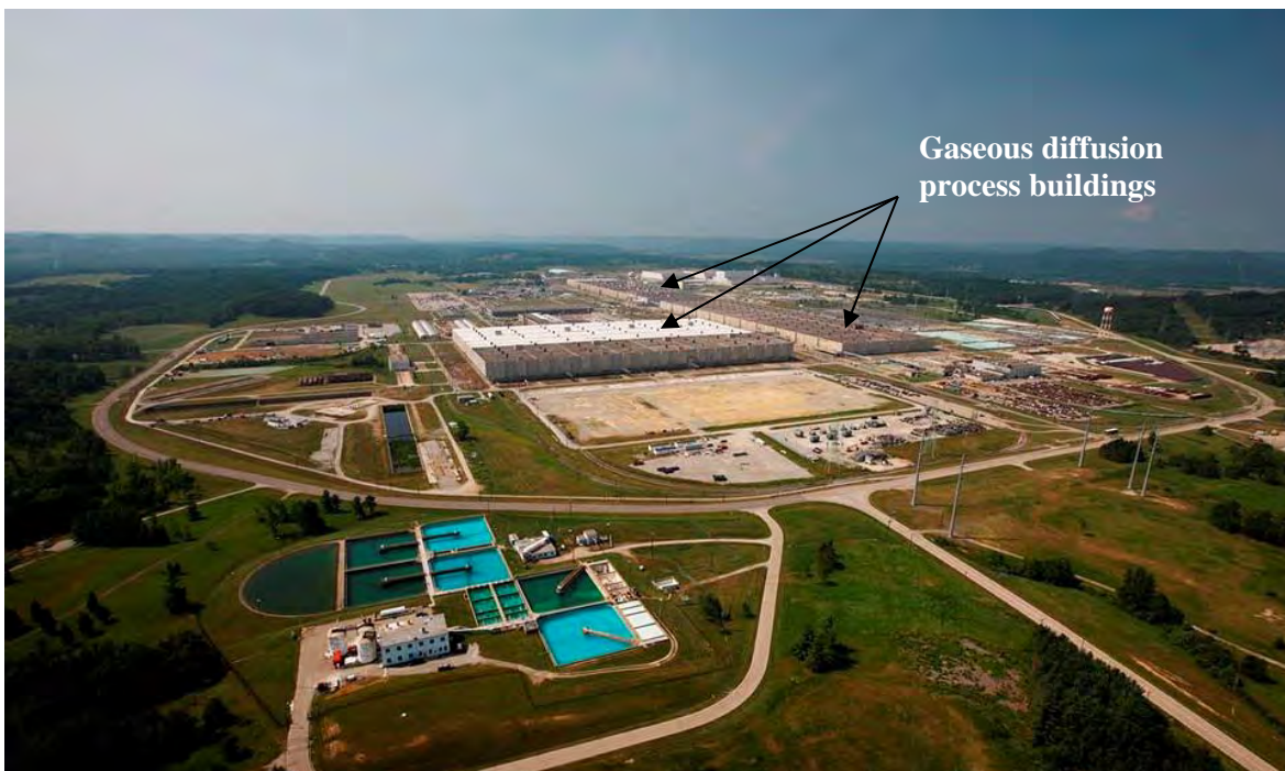
Figure 1.1 The Portsmouth Gaseous Diffusion Plant.
