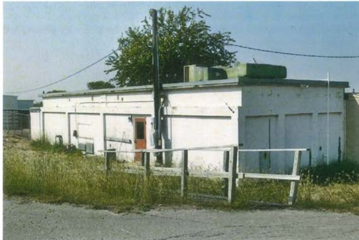
1. View of Building 91, facing south.
