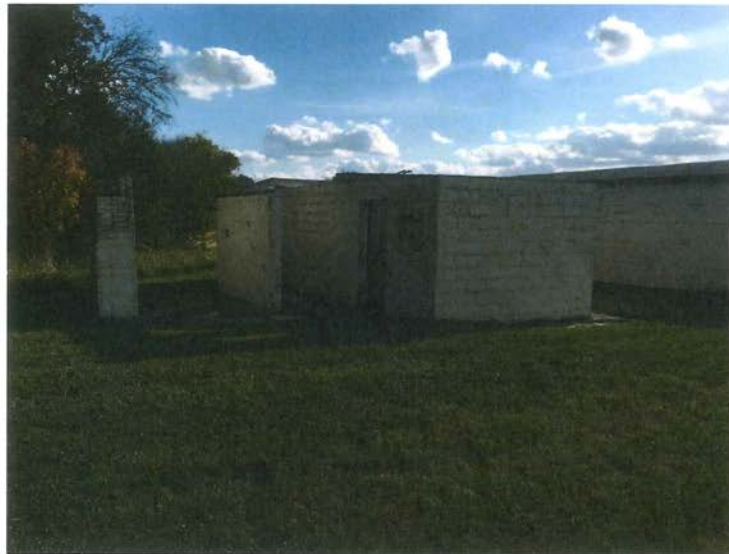
4. View of concrete block structure, facing south.
