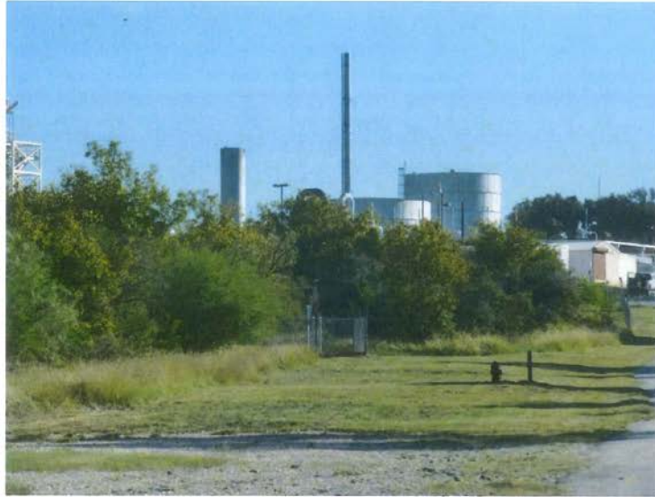
5. View from Avenue F Access Road, at southeast corner of facility site, facing east.
