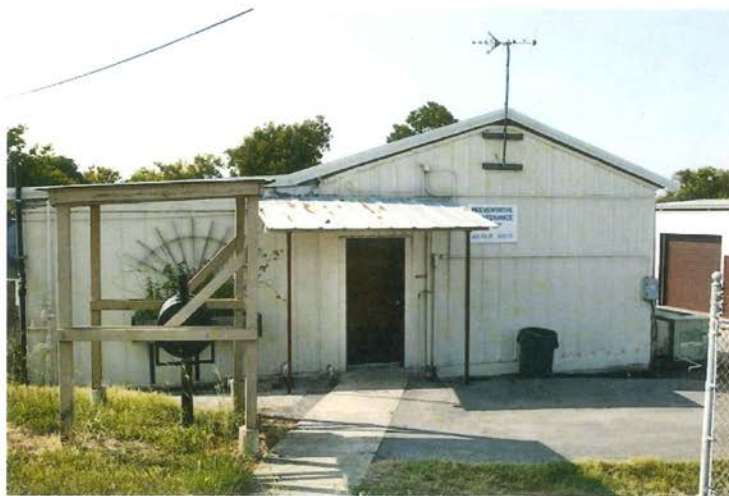
2. View of Building 112 facing south.
