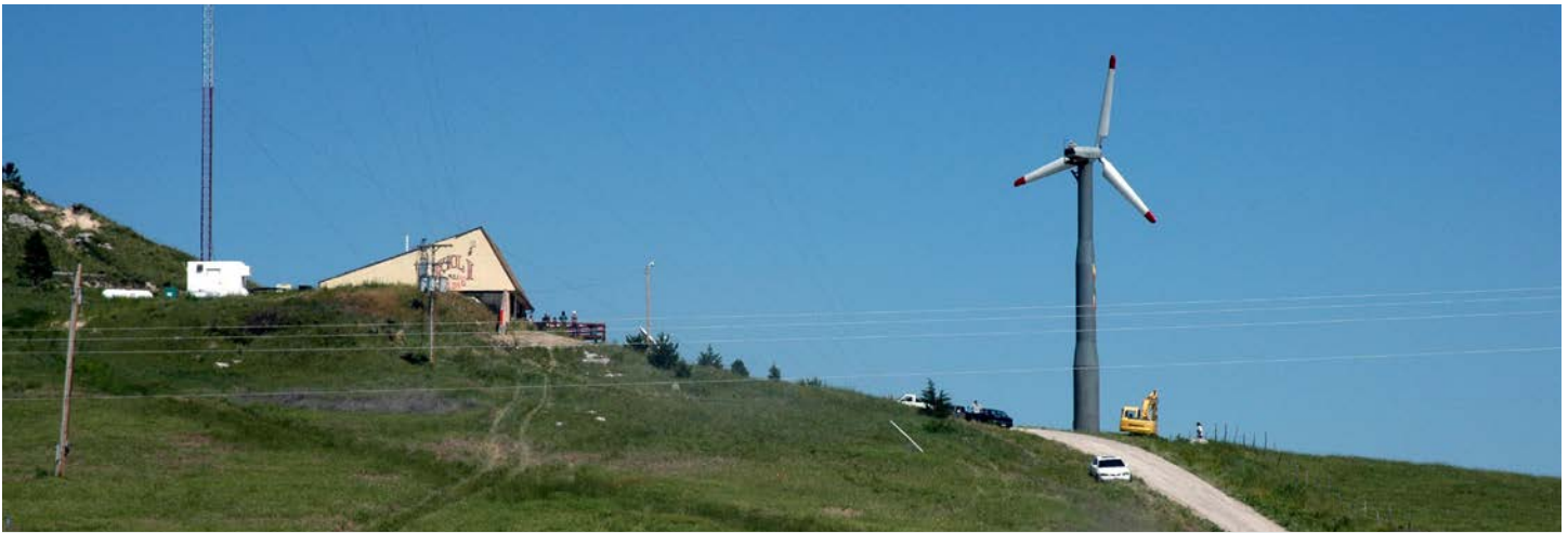
The Lakota Nation installed a 65-kW Nordtank turbine that annually supplies 120 MWh of power to KILI, the Pine Ridge Reservation radio station known as the voice of the Lakota Nation in South Dakota. Photo by Bob Gough, NREL 16258
