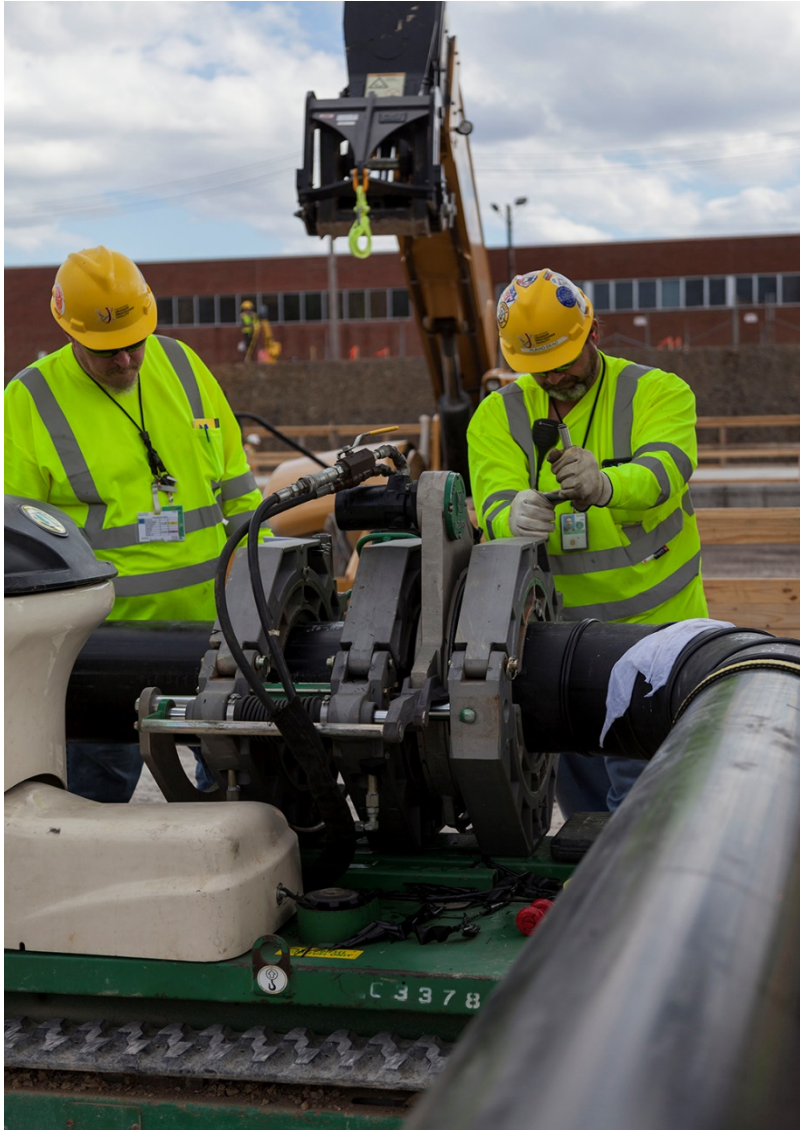
Potable Water Line Fusion Welding (MEB Subproject)
