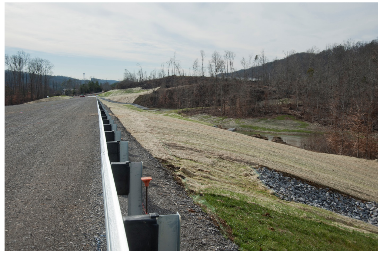
UPF Construction Haul Road
