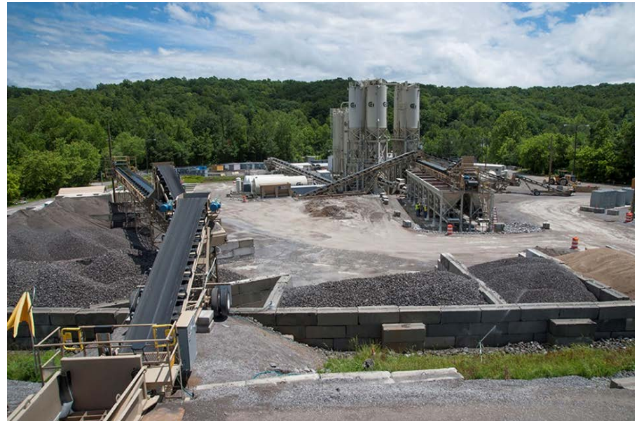
Concrete Batch Plant
