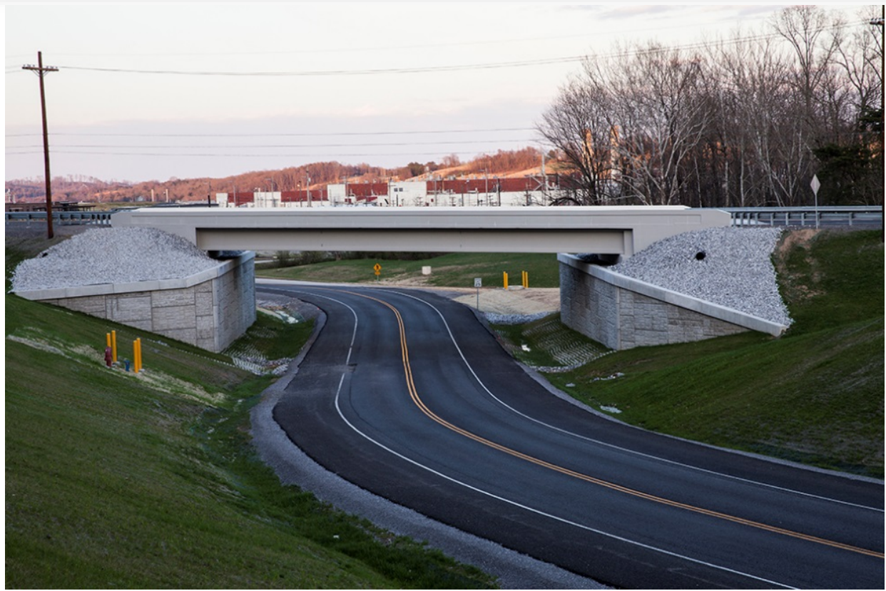
Bear Creek Road and Bridge
