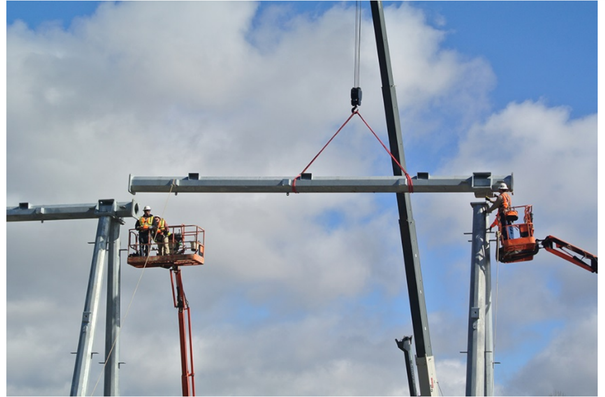
Erection of A-Frames (Substation Subproject)
