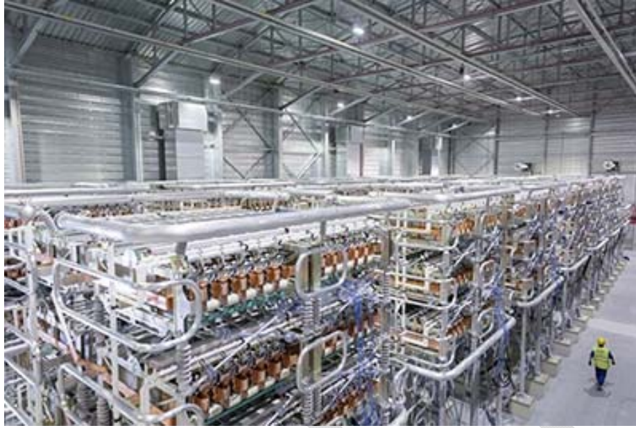
Figure 3: HVDC Converter Hall for 320 kV 2 GW VSC Transmission Link Between France and Spain
