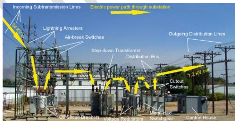
Figure 2: Power Flow and Equipment in a Distribution Substation 4
