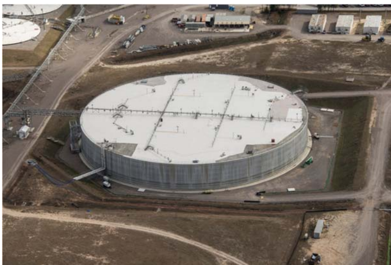
Photo 4: Completed Cell. 2017 U.S. Department of Energy Saltstone Disposal Unit 6, Savannah River Site.
