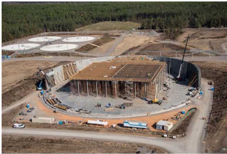
Photo 3: Construction Progress on Tapered Wall Sections and Reinforced Concrete Roof. 2017 U.S. Department of Energy Saltstone Disposal Unit 6, Savannah River Site.
