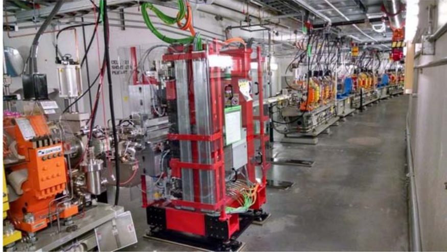
Photo 9: NEXT Elliptically Polarized Undulator Installed in Cell 21 of the NSLS-II Storage Ring Tunnel.
