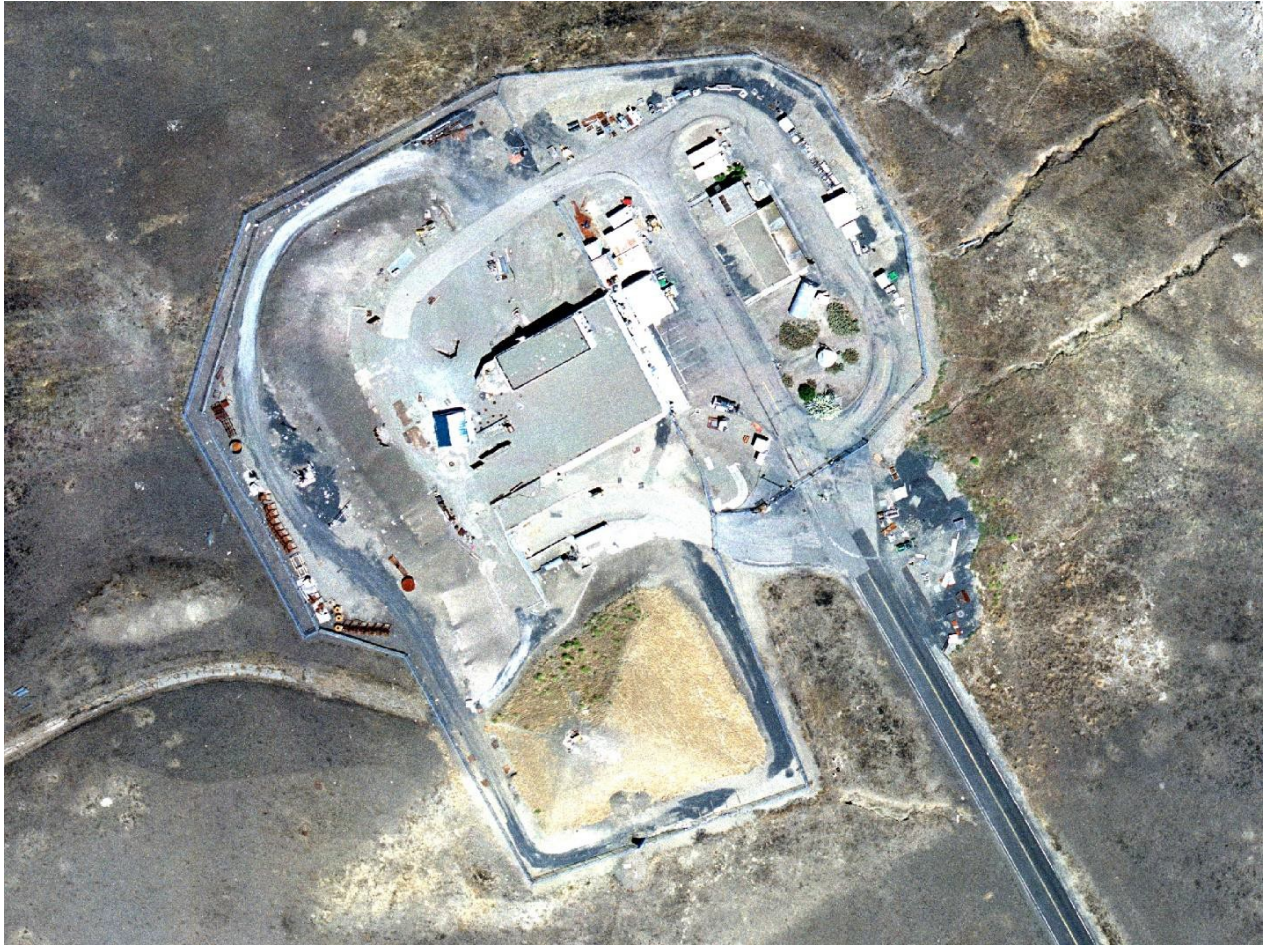
Figure 3. Aerial Photograph of the Building 851 Complex.
