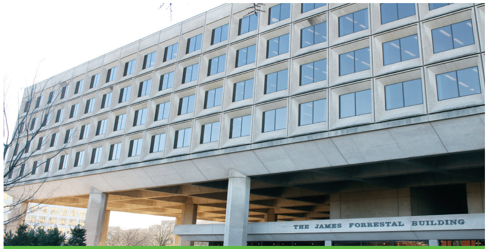
James Forrestal Building is the Department of Energy Headquarters. Photo credit Pacific Northwest National Laboratory.
