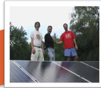
#5 Install Solar / PV
