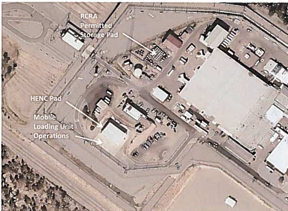
Figure 1. Location of the proposed mobile loading unit operations at TA-55
