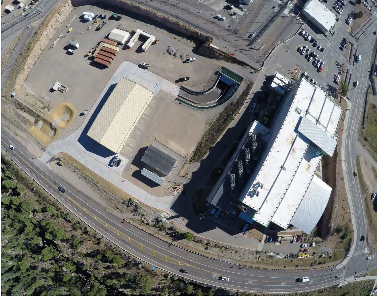
RLUOB site with Construction Access, Breakroom and Staging Area (2017)
