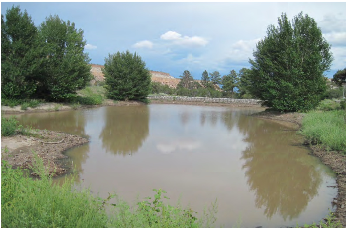
Figure 7-15 Los Alamos Canyon weir before (top photo) and after (bottom photo) storm-water flows
