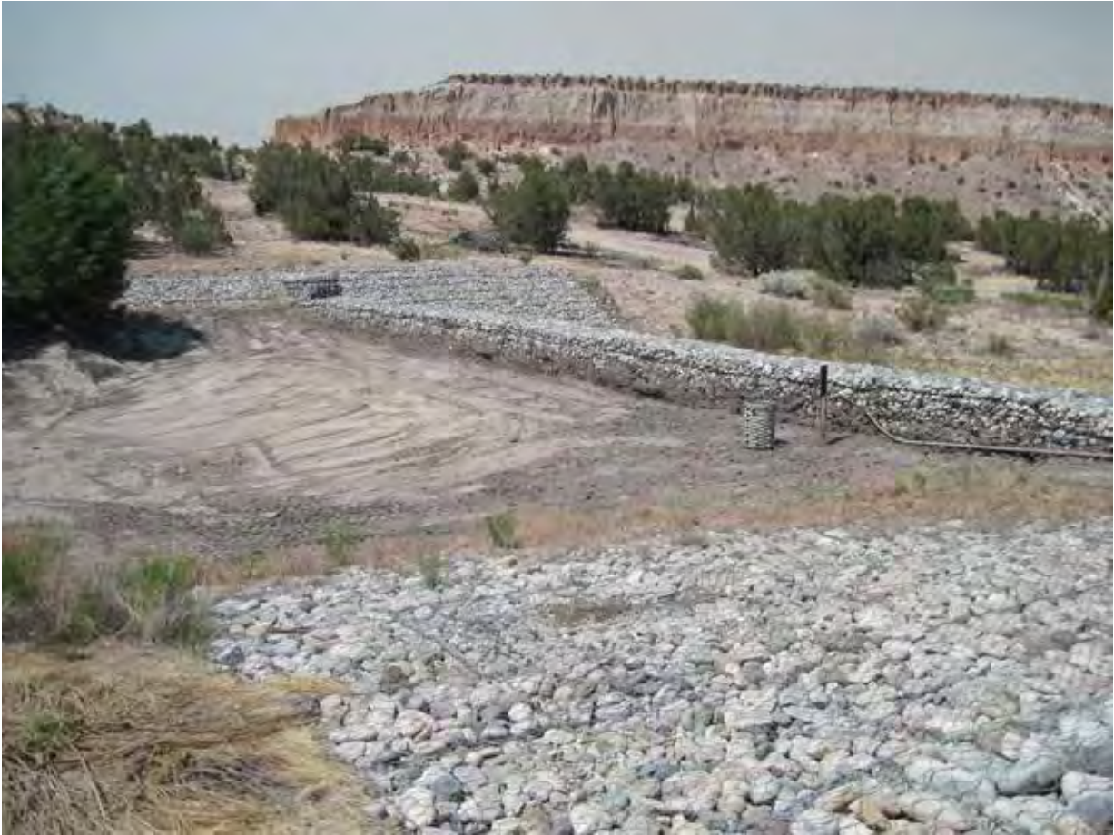
Figure 7-16 Los Alamos Canyon weir after sediment excavation in 2014
