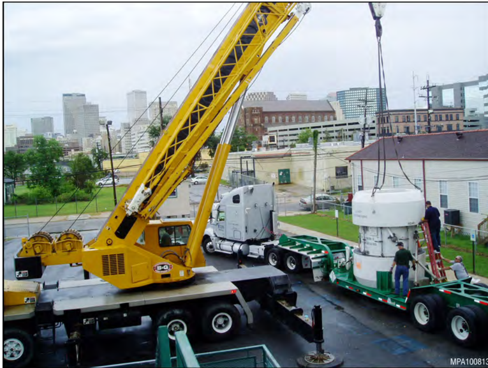
25 26 FIGURE 5.2.9-1 Transport of Radioactive Waste Containers 27
