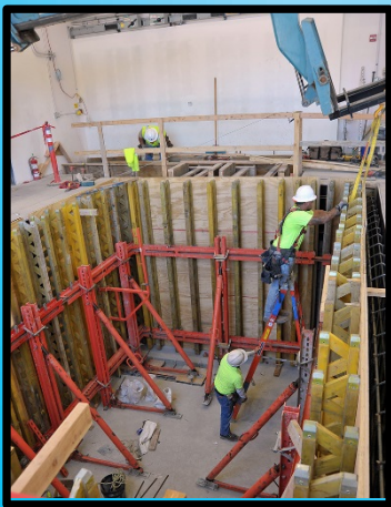
A crew from Summit Construction Co. of Albuquerque works on a project at Sandia National Laboratories
