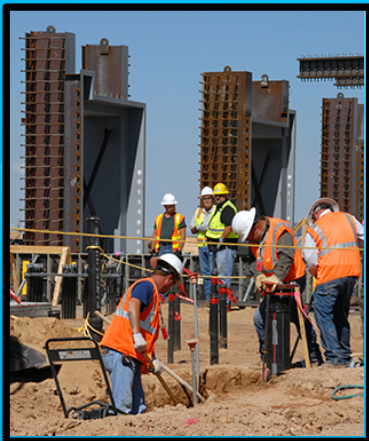
Construction of the High Explosives Pressing Facility at Pantex increased safety and aided production at the plant
