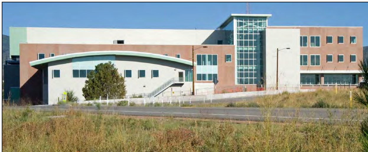
Figure 2-3 Radiological Laboratory/Utility/Office Building in Technical Area 55
