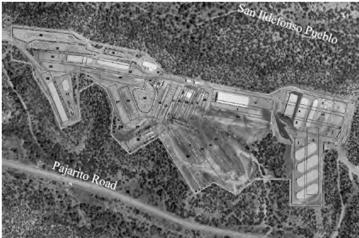
Figure I–15 Waste Management Areas within the Existing Area G Footprint in Technical Area 54
