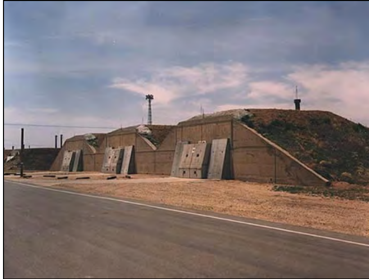
Figure 3.7-3—Typical Storage Igloos at Pantex
