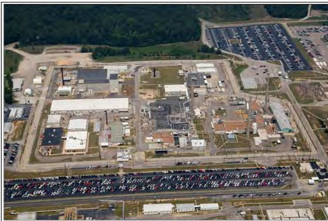
Figure A.7.1-3—Aerial Photo of SRS Tritium Facilities
