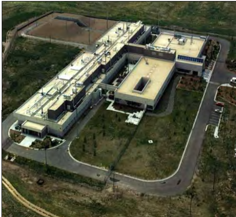
Figure A.6.1-6—Explosive Component Facility (ECF); SNL/NM Bldg 905
