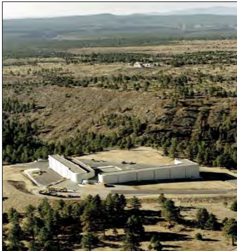
Figure A.9-4—The DARHT at LANL
