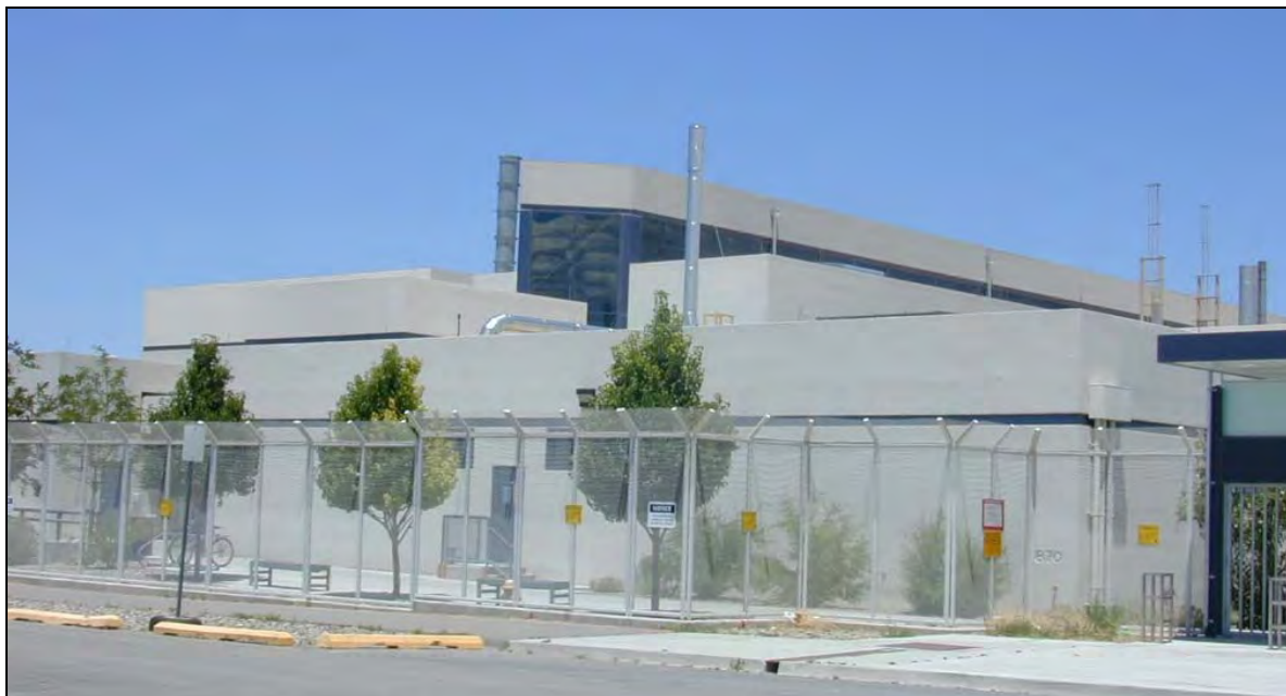
Figure A.7.1-4—Neutron Generator Production Facility at SNL/NM
