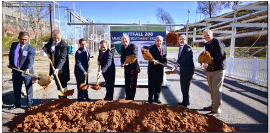
DOE, state and local officials break ground for the new Mercury Treatment Facility at Y-12.
