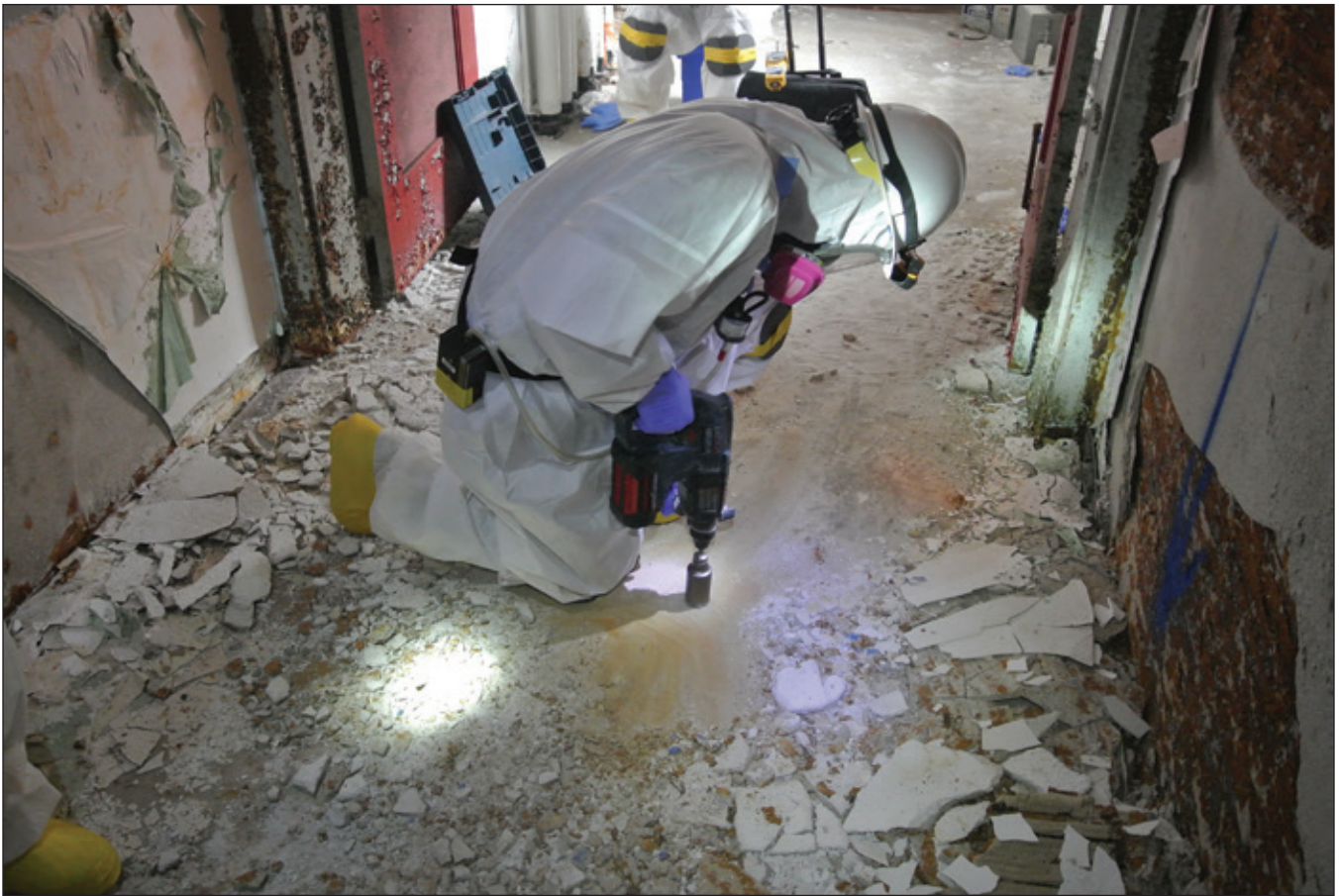
A worker takes a sample from a concrete floor in one of the Biology Complex facilities to determine the extent of contamination present
