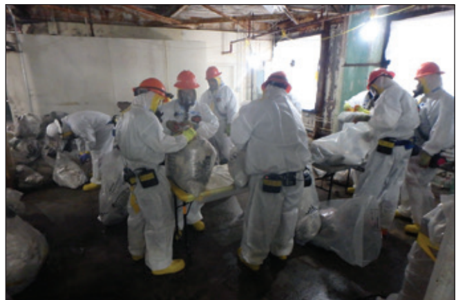
Asbestos abatement crew inside Building 7500
