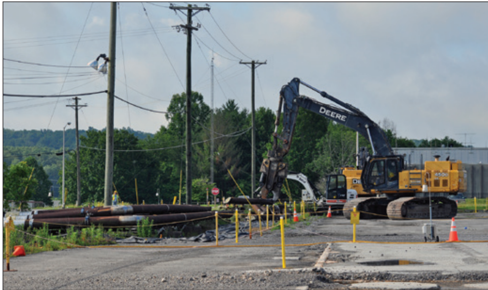
Demolition of the K-832 Cooling Water Pumphouse (above) and removal of tie lines (right).
