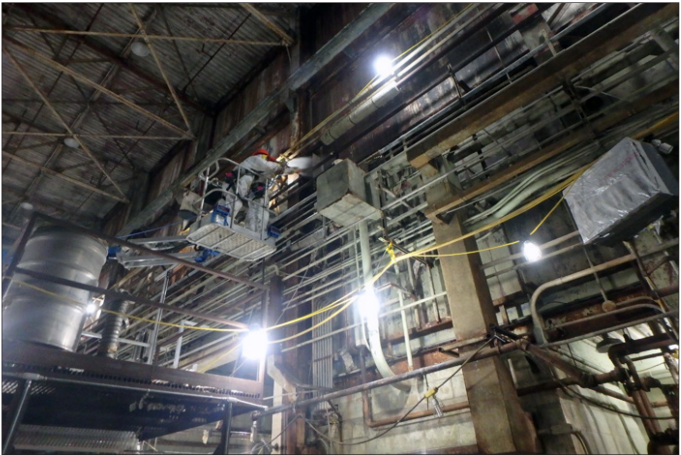
Asbestos removal in Building 7500
