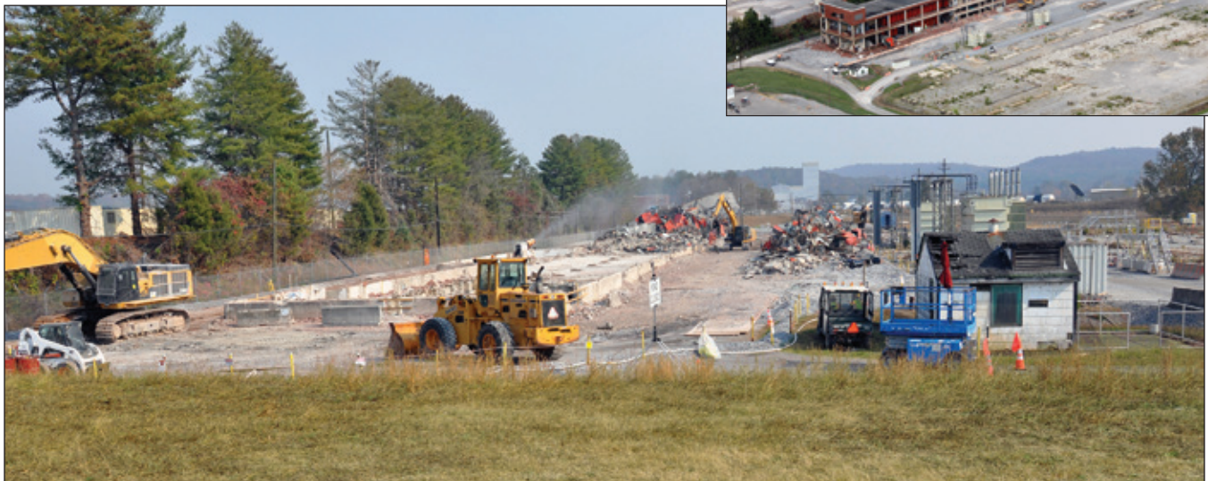
K-731 Building site after demolition
