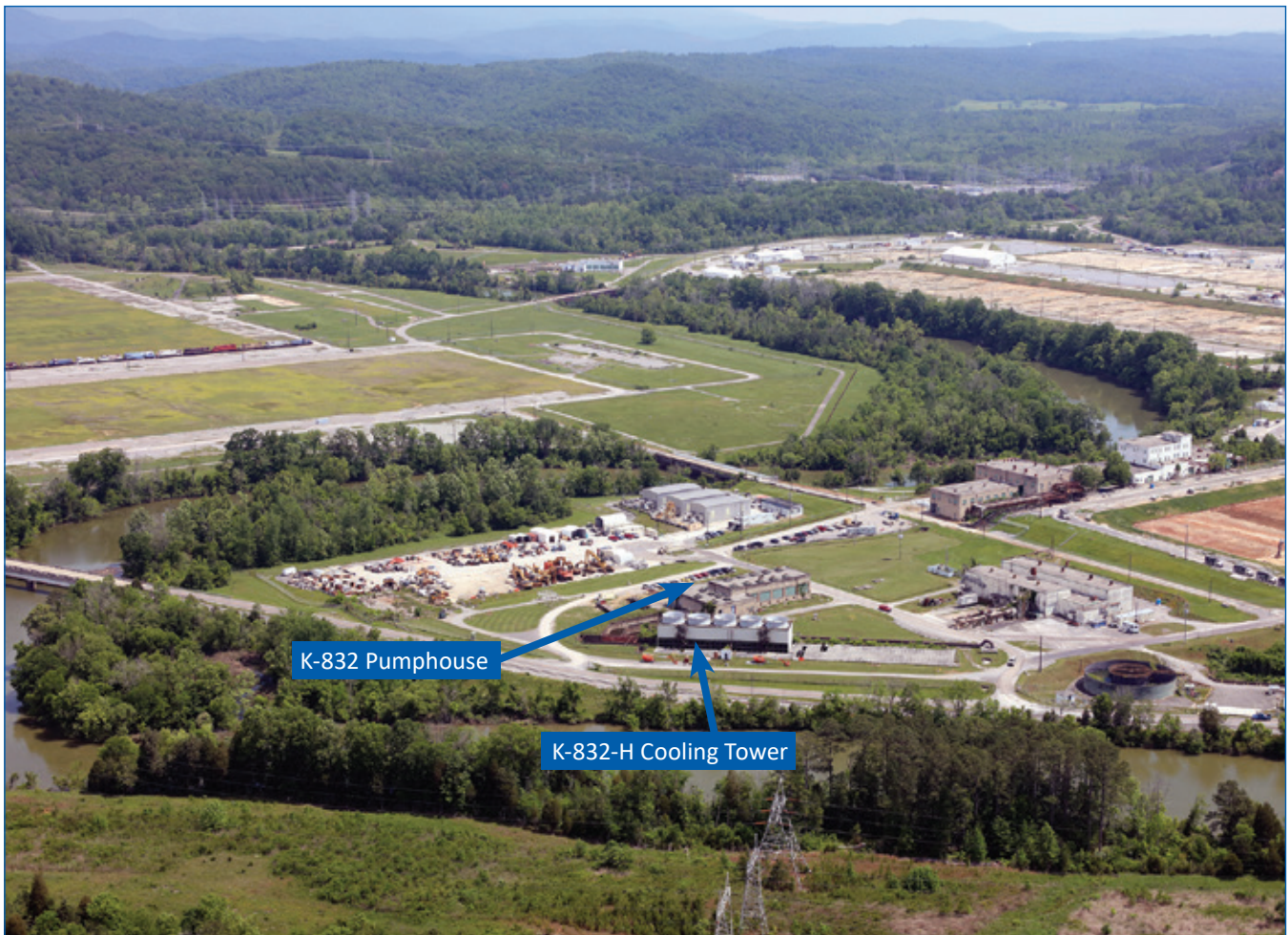
ETTP Poplar Creek area before demolition activities
