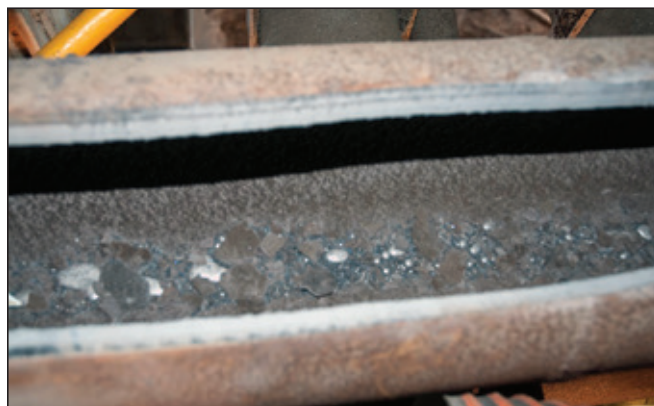
Some of the mercury-contaminated pipes contain a grit-like substance that requires a more aggressive technique to remove
