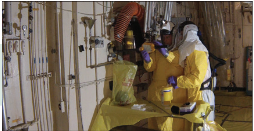
Fogging operations in Building 3029 hot cells
