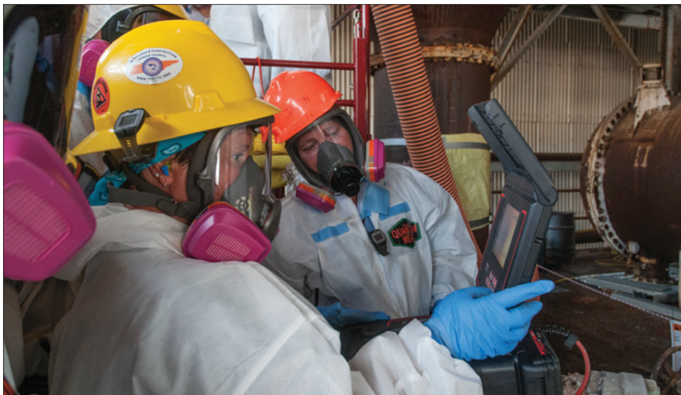
Workers use special equipment to view inside the COLEX equipment
