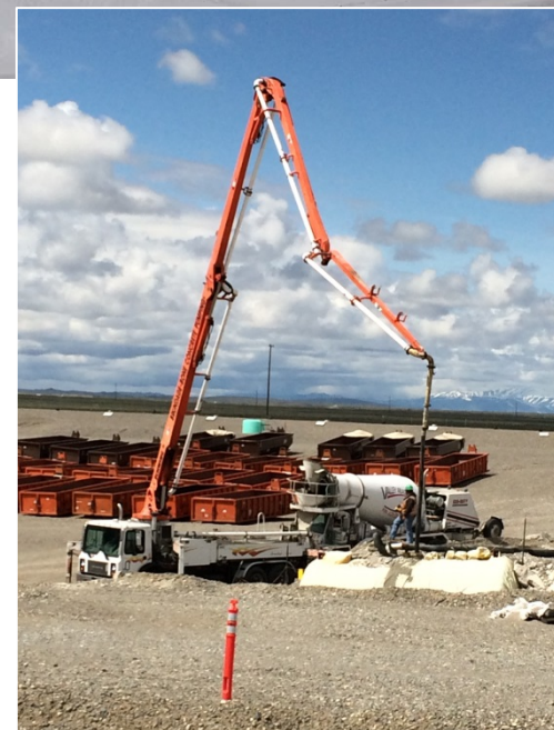
Grouting void spaces in legacy containers
