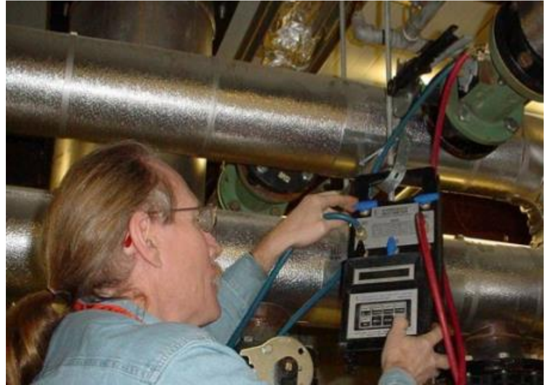
Verifying flow at a boiler
