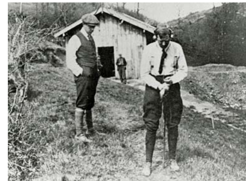
Conrad Schlumberger (1912) developing first wireline tool concept. Analog current injection.
