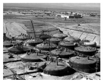
The Hanford Site's single-shell underground storage tank system was built from 1943–1964. The Draft EIS analyzes the potential environmental impacts of closure of Hanford's 149 single-shell tanks.
