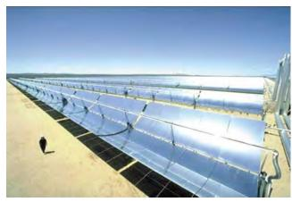
An example of a concentrating solar power U-shaped (parabolic) trough system at Kramer Junction, California.
