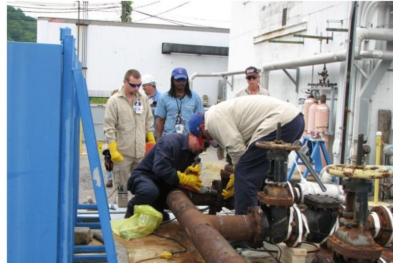
LGWO System Repairs
