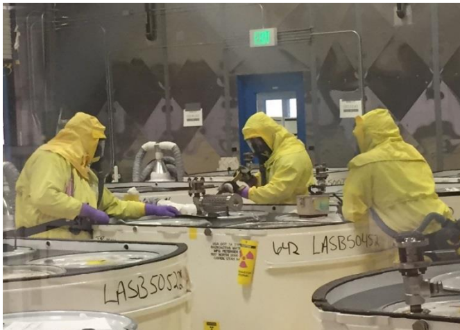
Workers installed pressure relief devices onto the lids of the RNS drums
