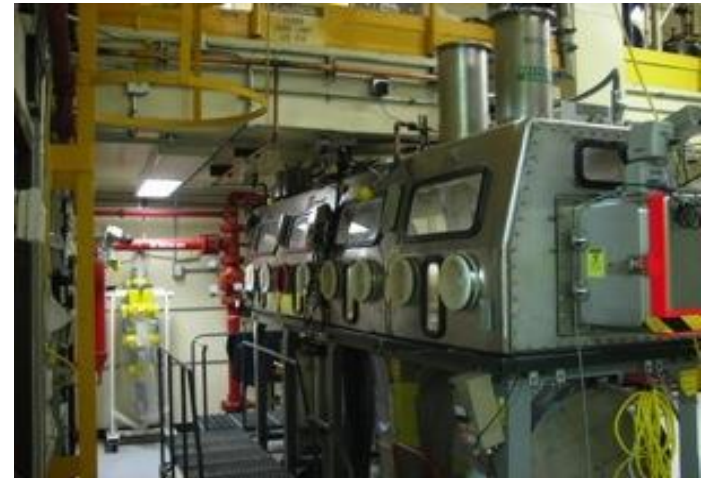
The glove box inside WCRRF underwent readiness reviews prior to the start of treatment
