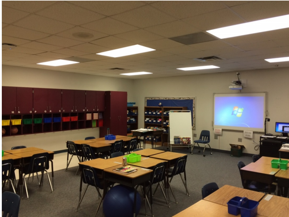
Figure 2. The reference classroom at Dale B. Davis Elementary School, with the incumbent nine-luminaire fluorescent lighting system.
