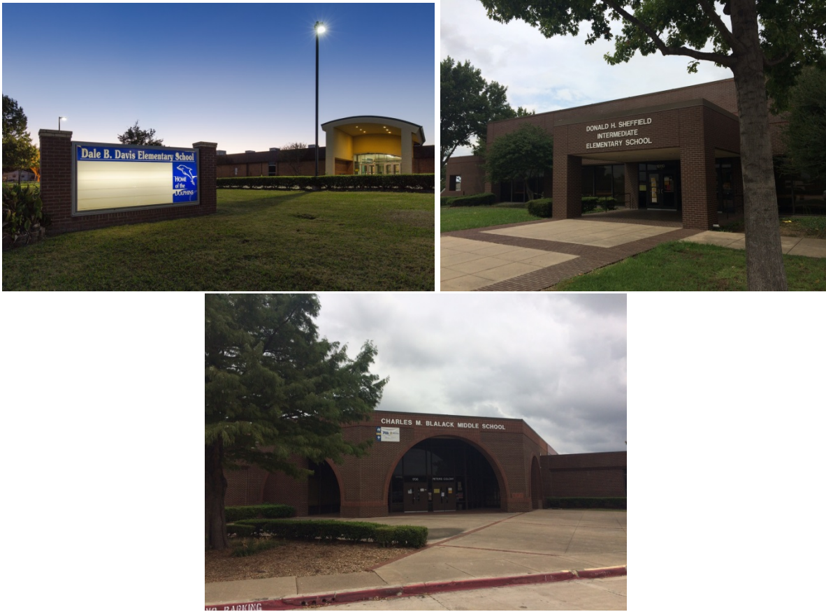
Figure 1. Exterior view of the three schools in the Carrollton-Farmers Branch Independent School District that participated in the LED lighting system installation and evaluation project. One classroom in each school was outfitted with a new lighting system. (Credits: ABL for DES, PNNL for others.)
