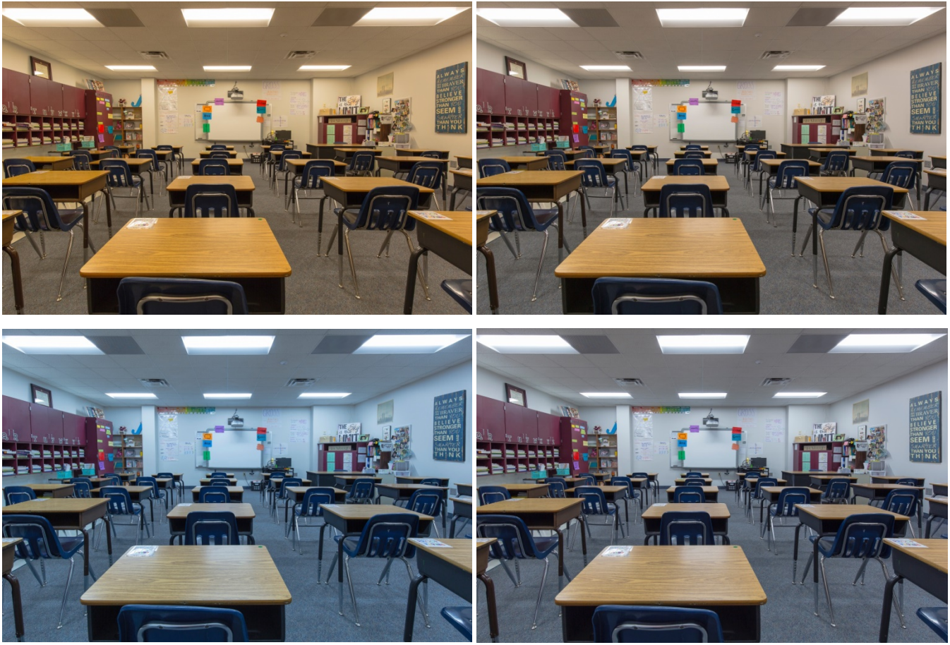
Figure 5. New tunable lighting in the classroom at DES. The four SPD settings are shown in clockwise order, beginning with the upper left photo: 3000 K (Reading), 3500 K (Testing), 4200 K (General), and 5000 K (Energy). The Scene 1 setting was used during the photographs, so all luminaires were on at full light output. (Photos courtesy of ABL.)
