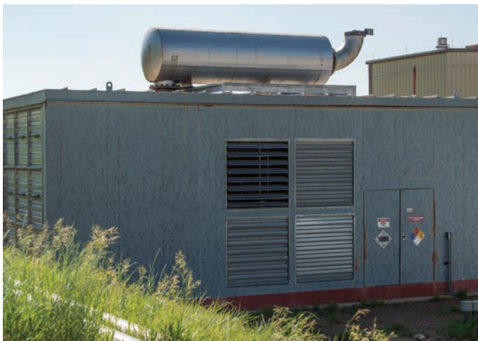
A double-wall 500-gallon (1,893-liter) diesel fuel tank is located inside this standby generator enclosure at the Integrated Biorefinery Facility. Photo by Dennis Schroeder, NREL 45424
