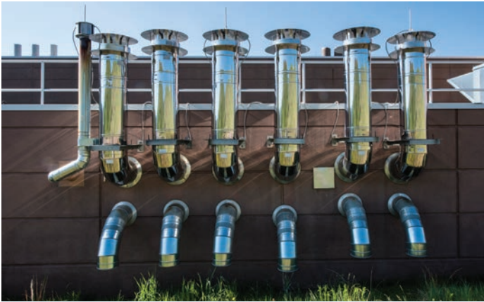
Air inlets and exhaust stacks for six natural-gas-fired, low-NO x -emitting hot water boilers which provide comfort heating to the Field Test Laboratory Building. Photo by Dennis Schroeder, NREL 45415
