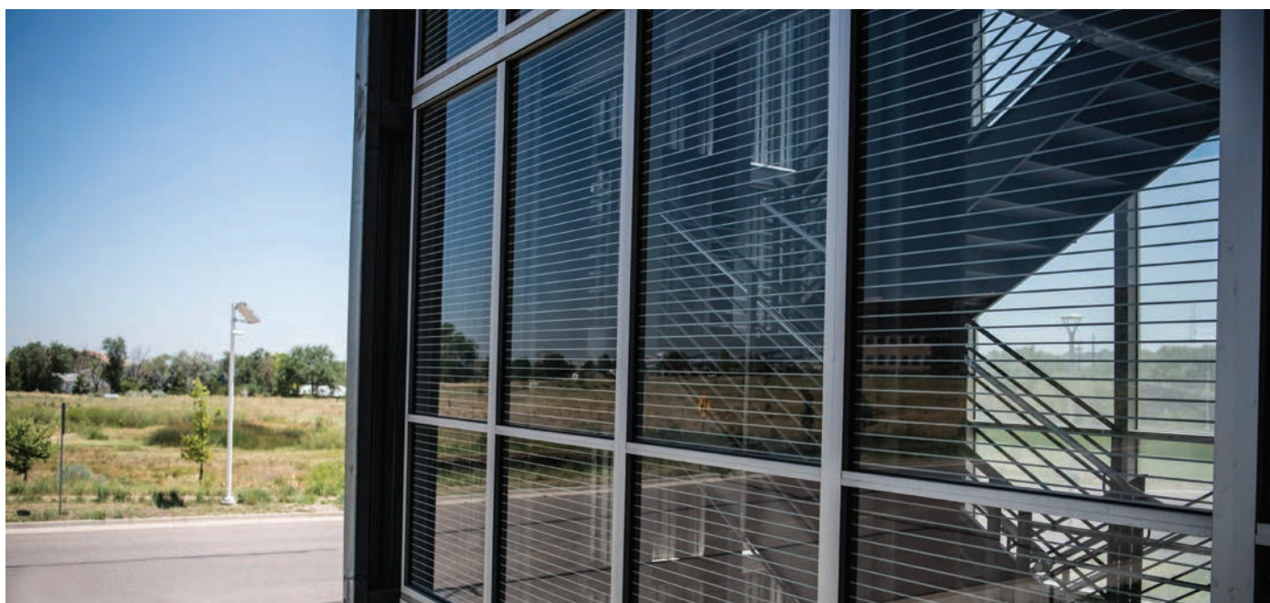
Special fitted glass was installed on stairwell enclosures at the STM site employee parking garage to prevent bird collisions, a major cause of avian mortality, by making the glass more visible to them. Photo by Dennis Schroeder, NREL 46044
