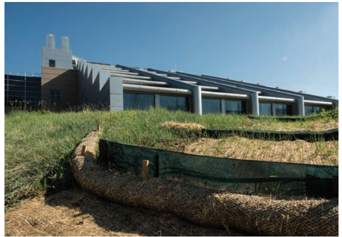
Erosion control measures protect native seed sown into an area disturbed during a culvert repair project at the STM site. Photo by Dennis Schroeder, NREL 45409
